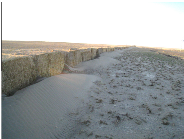
Fig. 9. Wind-blown sediment trapped behind straw bales protecting a county road downwind of the burned area in early April 2011, 8 months after the fire.
