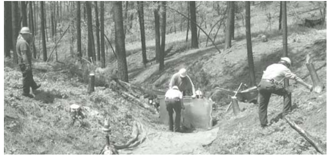
Figure 1. Sheet metal cut-off wall installation.
