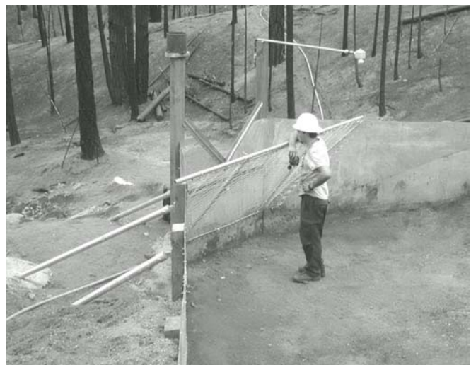
Figure 3. V-notch weir and trash/debris screen.
