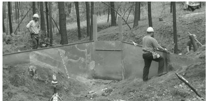
Figure 2. Sidewalls of sediment trap.
