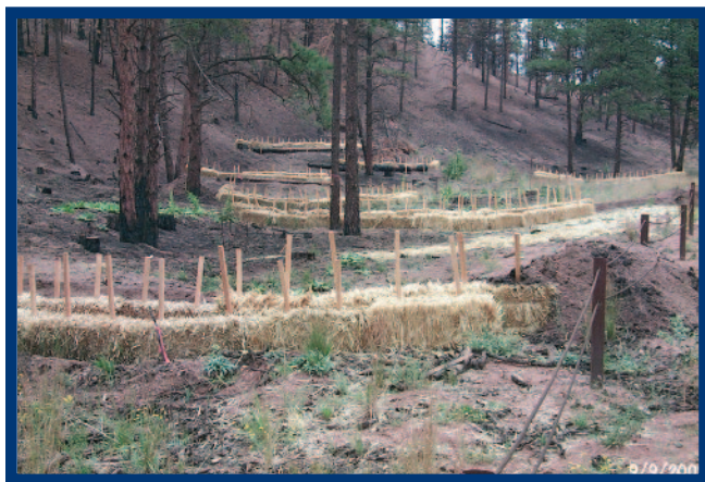
Figure 10.3 —Straw bale check dams placed in channel by the Denver Water Board after the Hayman Fire, 2002, near Deckers, CO. (Photo by Peter Robichaud).
