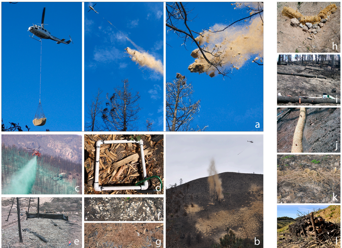
Fig. 5. Photographs of common ground cover and barrier treatments included in the meta-analysis: a) straw bale transport by helicopter (2005 School Fire, Washington, USA); b) helimulching dropping (2015, Navia de Suarna, Lugo, Spain); c) aerial hydromulch application (2002 Hayman Fire, Colorado, USA); d) wood shred mulching ground cover frame (2012 Waldo Canyon Fire, Colorado, USA); e) wood strand mulch study plot (2002 Hayman Fire, Colorado, USA); f) wood chips mulch (2006, Soutelo de Montes, Pontevedra, Spain); g) bark strand mulch (2010, Fial das Corzas, Pontevedra, Spain); h) straw bale check dams in an ephemeral channel (2010 Twitchell Canyon Fire, Utah, USA); i) log barriers (2002 Canyon Fire, California, USA); j) straw wattle barrier (2000 Bitterroot Complex Fire, Montana, USA); k) barriers made with shrubs (2006, Soutelo de Montes, Pontevedra, Spain); l) log dam (2015, Cinco Villas, Orés, Spain).
