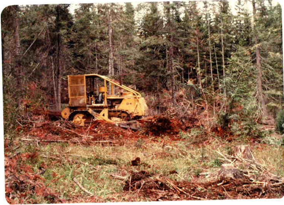
Figure 4. Redistribution of soil due to vertical placement of the dozer blade.
