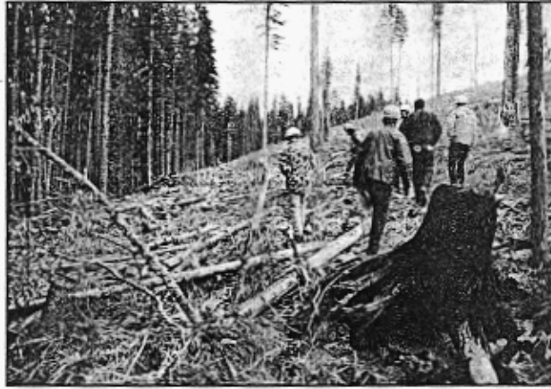
Recontoured road which will successfully eliminate surface hydrologic and erosion problems, but which may lead to slope failure or gullying because of a major seepage line along the base of the former cutslope some 3 m. below the surface.
