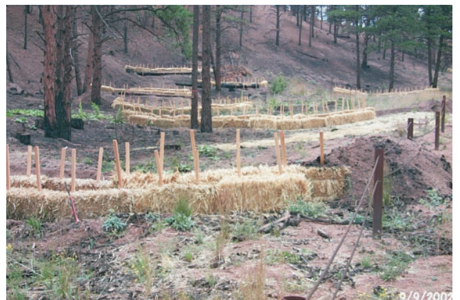
Figure 14 —Strawbale check dams located on Denver Water Board property within the Hayman Fire area.
