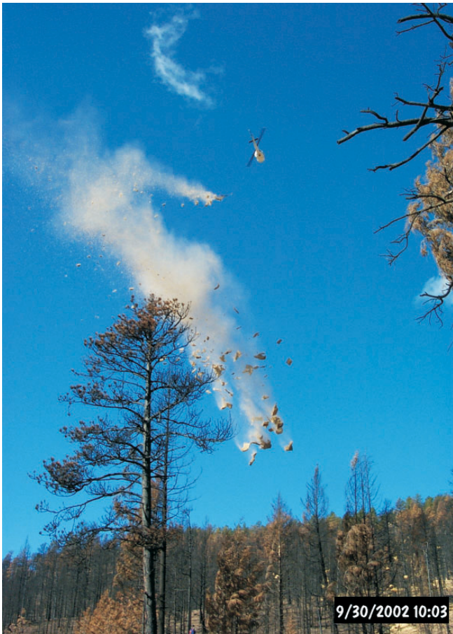
Figure 11 —Aerial dry mulch being applied.
