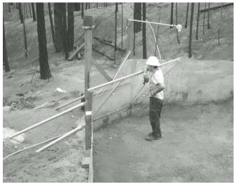
Figure 3. V-notch weir and trash/debris screen.
