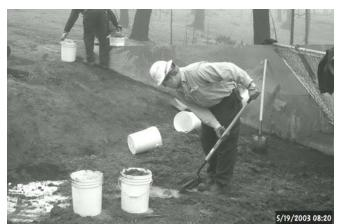
Figure 4. Buckets are used for sediment clean out.
