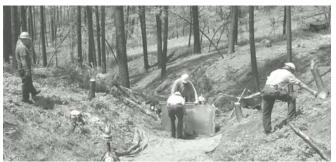
Figure 1. Sheet metal cut-off wall installation.
