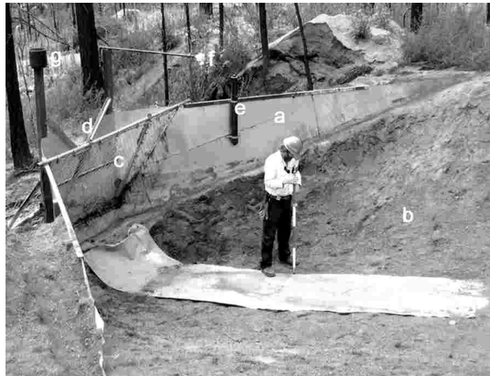
Figure 1. Typical paired catchment sediment basin after removal of sediment. a) sheet metal barrier wall; b) sediment basin area; c) debris collection rack; d) V-notch weir; e) magnetic/electronic stage sensor; f) ultrasonic depth sensor; g) tipping bucket rain gauge (Robichaud 2005).
