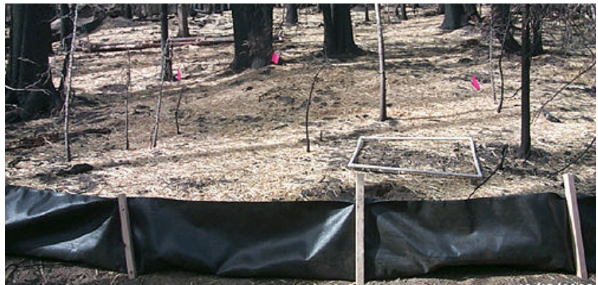
Silt fence installation and completion, after the 2003 Hot Creek fire, James Creek, Atlanta -- comparing to the effectiveness of straw mulch.
